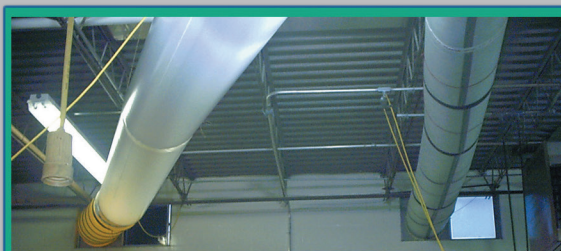
Temporary Air Duct Distribution System
