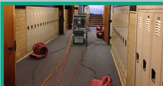
Electrical Distribution for Air Movers/110 Volt DH's
